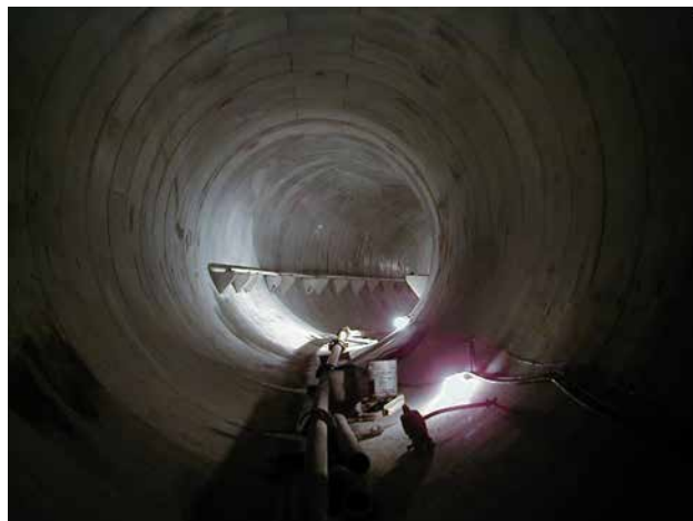
Above: Market Street shaft Left: Drainage construction workers
