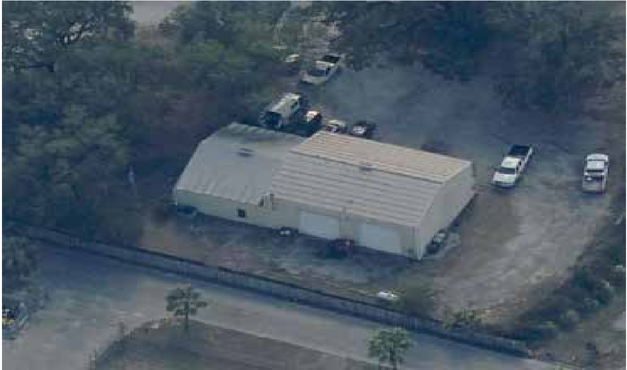
Current Fire Station 20
