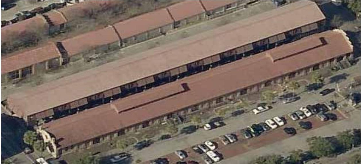
Visitors Reception and Transportation Center (VRTC)
