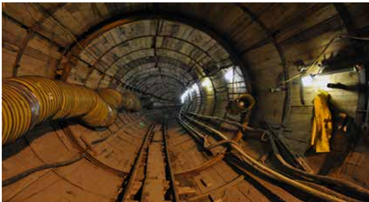
Market Street Drainage Tunnel
