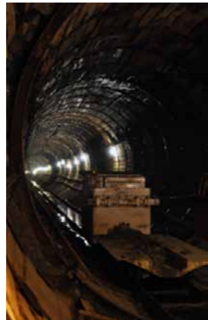
Charleston drainage shaft
