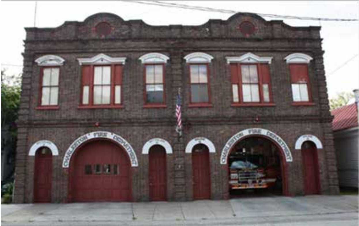
CFD Cannon Street Fire Station (FS 6)
