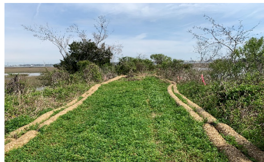
Construction photos provided by Capital Projects
