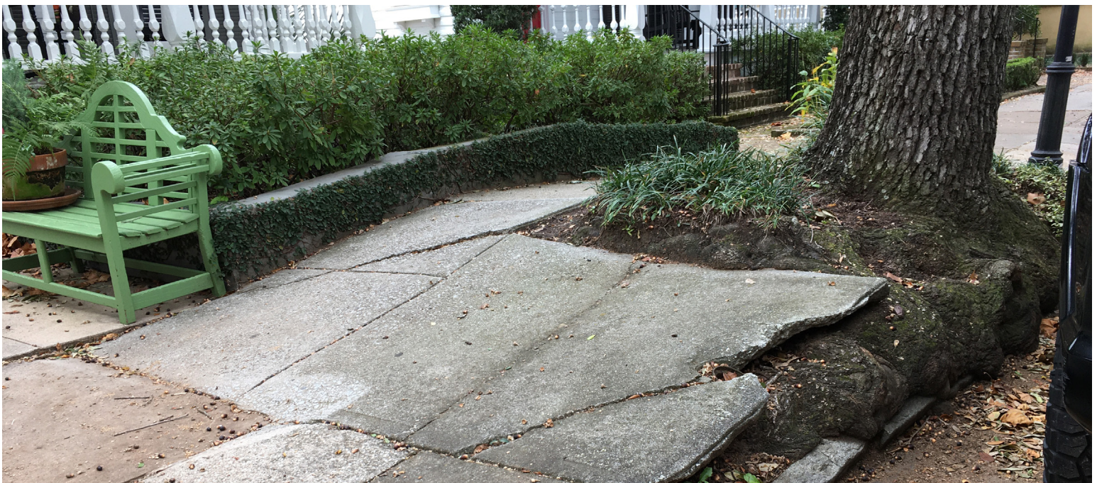
Typical tree root damage at a sidewalk.
