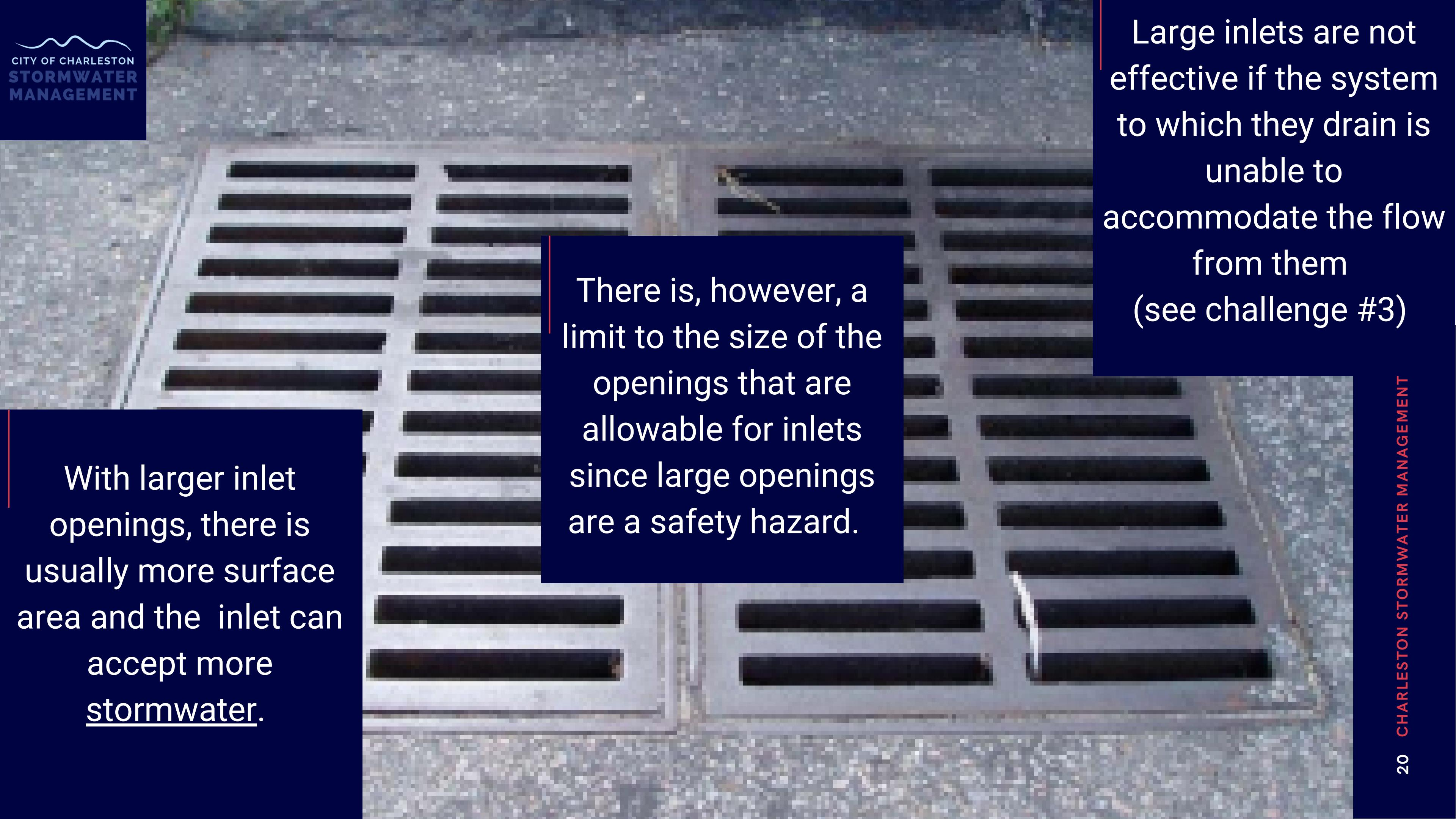
With larger inlet openings, there is usually more surface area and the inlet can accept more stormwater.
