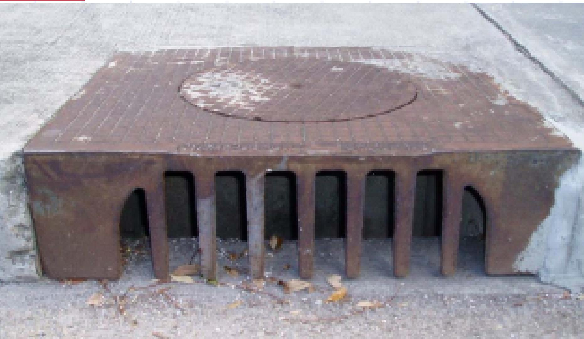
The number and size of inlets will affect how quickly an area can drain.
