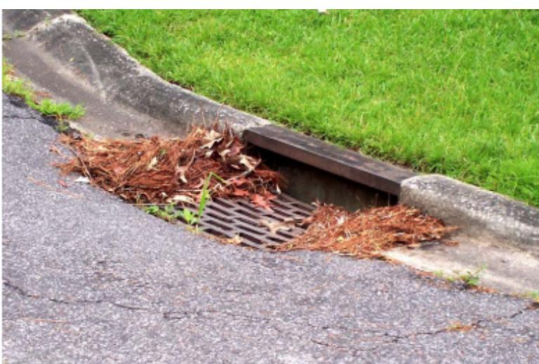
Trash and debris that gets caught on and in storm grates causes ponding to form on our ground surfaces, which leads to flooding.
