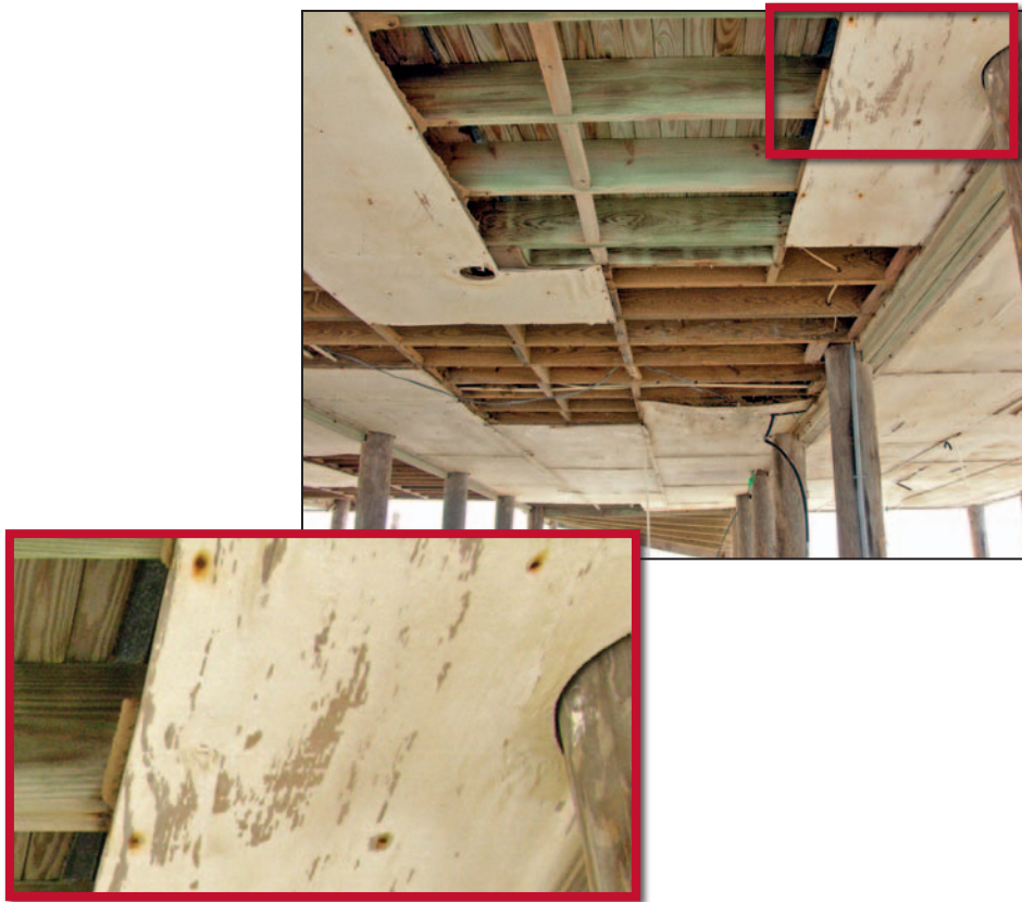
Figure 11-4. Plywood panels on the underside of a house that blew away because of excessive nail spacing. Note the corroded nails (inset). Estimated wind speed: 105 to 115 mph. Hurricane Ivan (Alabama, 2004)
