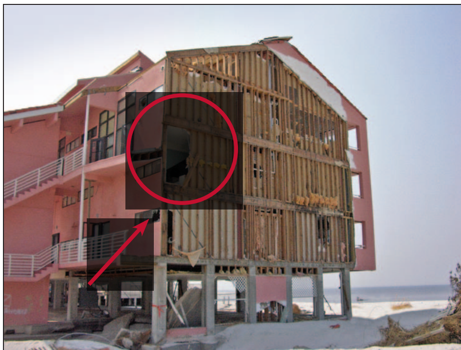
Figure 11-19. Blown-off EIFS, resulting in extensive interior water damage; detachment of the gypsum board or stud blow off (circle); two windows broken by debris (arrow). Estimated wind speed: 105 to 115 mph. Hurricane Ivan (Florida, 2004)
