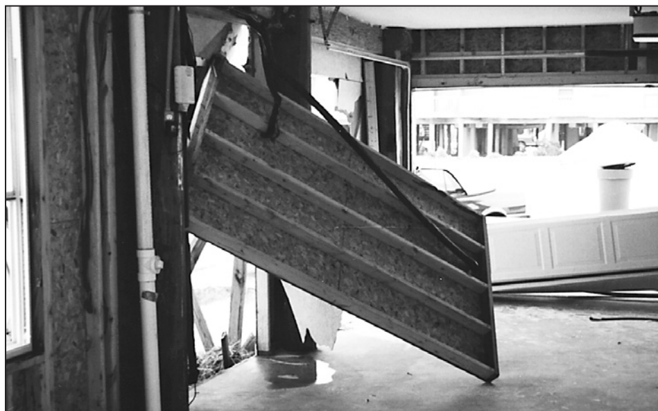
Figure 9-29. Breakaway wall panel prevented from breaking away cleanly by utility penetrations, Hurricane Opal (Florida, 1995)
