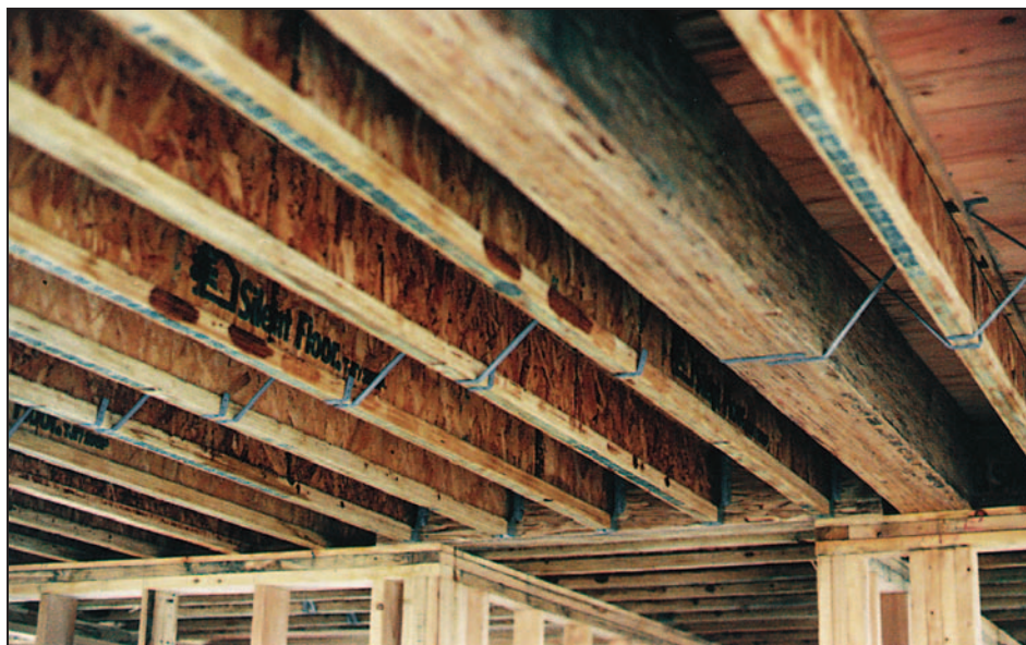
Figure 13-20. Engineered joists used as floor joists with proper metal brace to keep the bottoms of the joists from twisting; engineered wood beam
