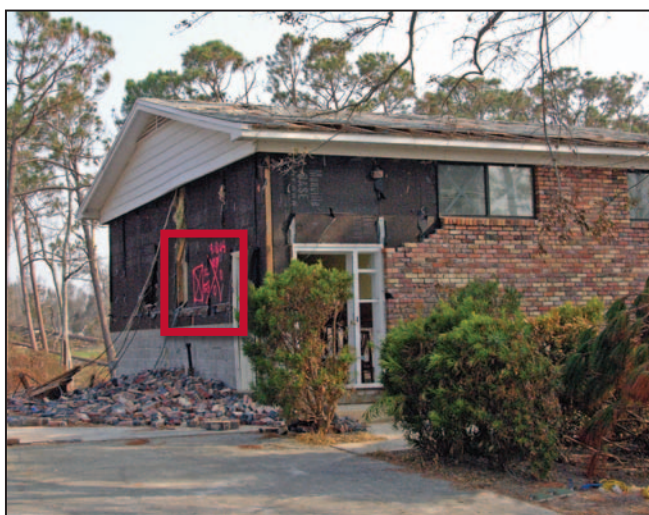
Figure 11-17. Four brick veneer failure modes; five corrugated ties that were not embedded in the mortar joints (inset). Hurricane Ivan (Florida, 2004)
