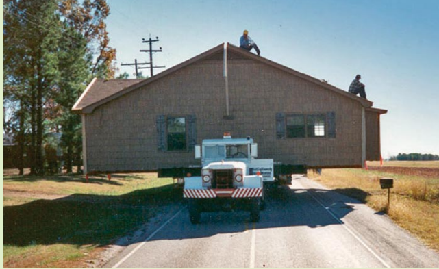
Hollis Kennedy House Movers
