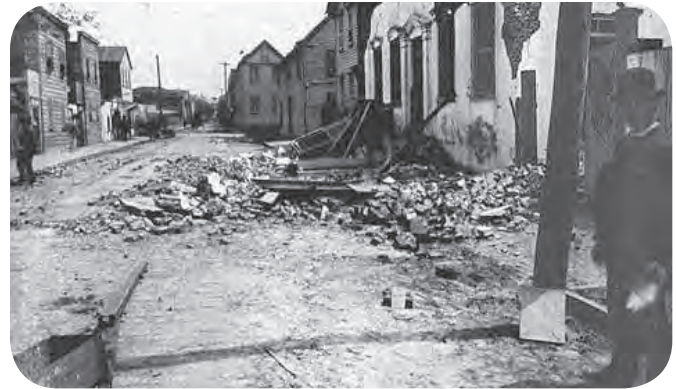
▲ Damage from the earthquake of 1886 ( http://www.eas.slu.edu/eqc/eqc_photos/1886EQ/sldjpgs/SLD19.html )
