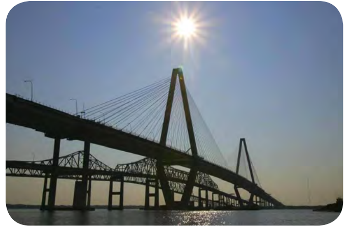
▲ Arthur Ravenel Jr. Bridge in 2005 before completion (TheState.com, Erik Campos)
