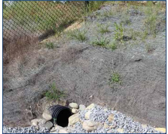
Figure 6. Steep slopes and exposed soils along this bank resulted in erosion and gullying, which can attribute to sedimentation in downstream best management practices like bioretention cells. Owners took action to repair this site by seeding the area with grass to stabilize, and installing an erosion control blanket to provide protection until grass establishes.
