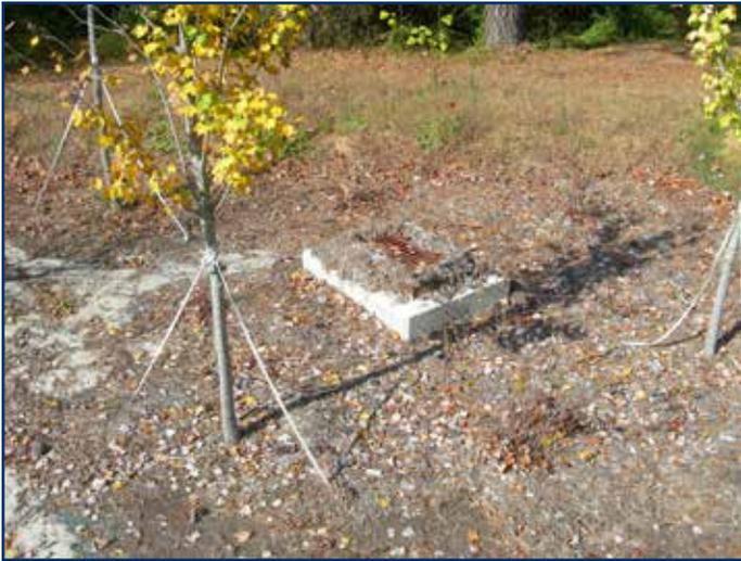
Figure 5. Without action to remove debris in the grate and cell, this grate may become clogged with floatable leaf litter and result in drainage problems in the bioretention cell. A new hardwood mulch layer should be established in the cell to prevent clogging, reduce exposed soils and minimize the chance of erosion. Photo courtesy Bill Lord, NCSU.
