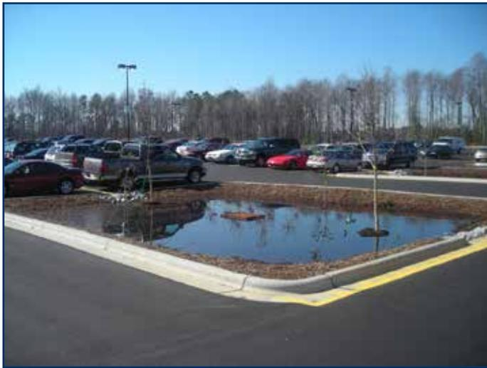
Figure 4. This parking lot bioretention cell has standing water outside of the recommended time to drain, an indicator that the cell may be clogged. Photo courtesy Bill Lord, NC State University.
